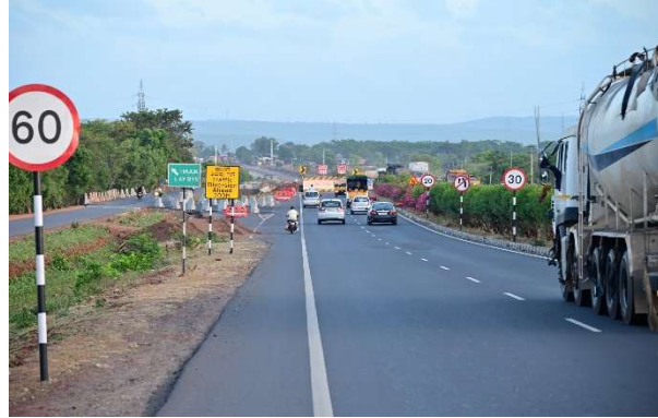
Road Diversion in Day Time
