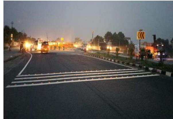
Road Diversion in the night
